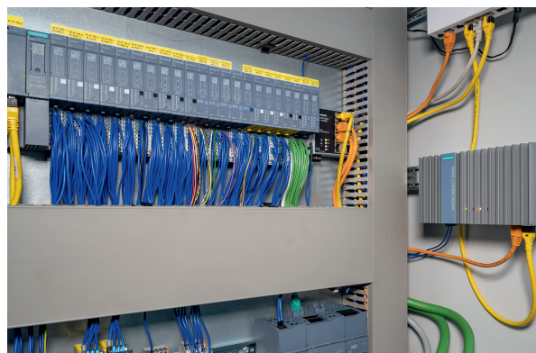
Fig. 4. Control cabinet: the compact Open Controller (left) integrates the functions of a PC-based, fail-safe software controller. Secure data transfer between the machine and the cloud-based software system MindSphere is realized by a MindConnect Nano-Device (right) © Siemens
