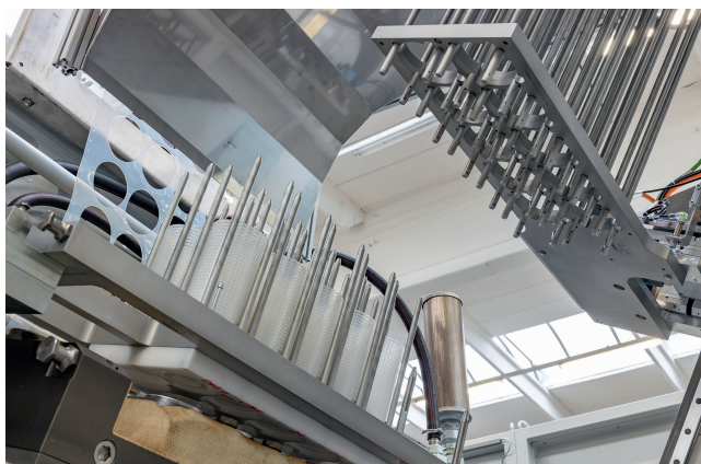
Fig. 2. A Simatic ET 200SP Open Controller from Siemens coordinates the interaction of all components in the thermoforming machine © Siemens
